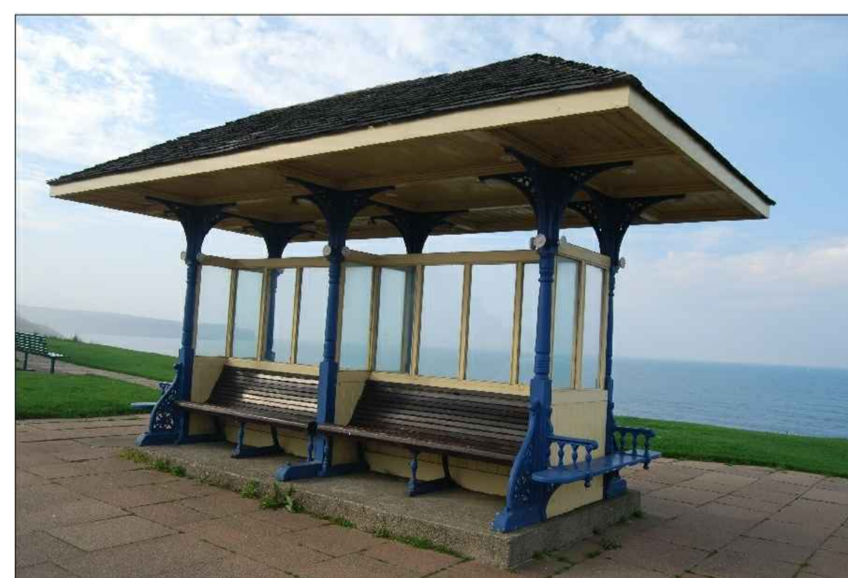
Edwardian Shelter to west of Cliff Lift, Promenade, Whitby Sep 2014 (One of an identical pair) Grade II EH List Entry No: 1389285
